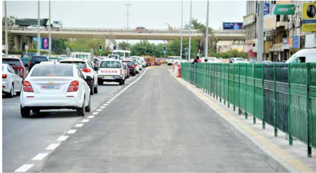
The major project aims to alleviate traffic congestion on Budaiya Highway
