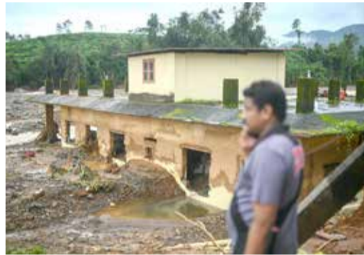
A man stands near a damaged house
