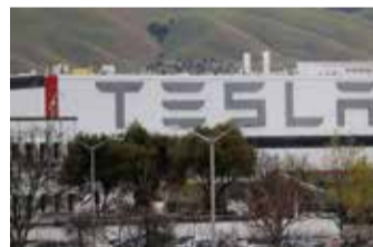
The view of Tesla Inc's US vehicle factory in Fremont, California
