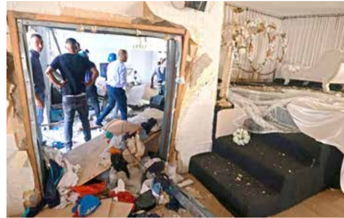
Palestinians inspect the damage following an Israel military raid in the occupied West Bank village of Al-Aqaba
