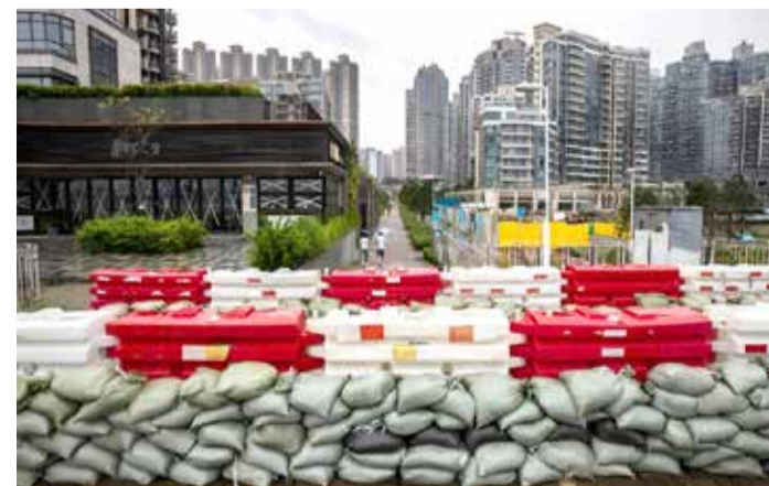
Sand bags are placed to stop flooding by the waterfront at Tseung Kwan O in Hong Kong
