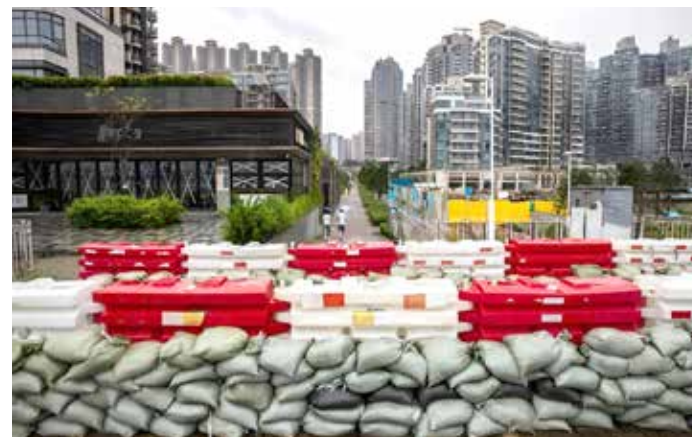
Sand bags are placed to stop flooding by the waterfront at Tseung Kwan O in Hong Kong
