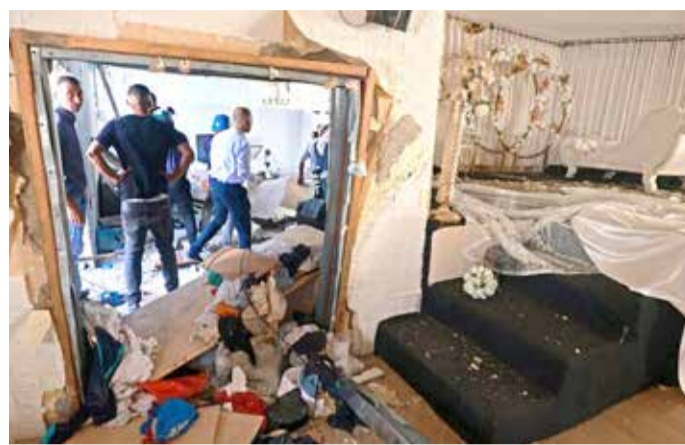
Palestinians inspect the damage following an Israel military raid in the occupied West Bank village of Al-Aqaba
