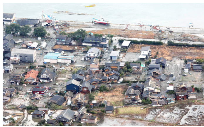
damage in the city of Suzu, Ishikawa prefecture
