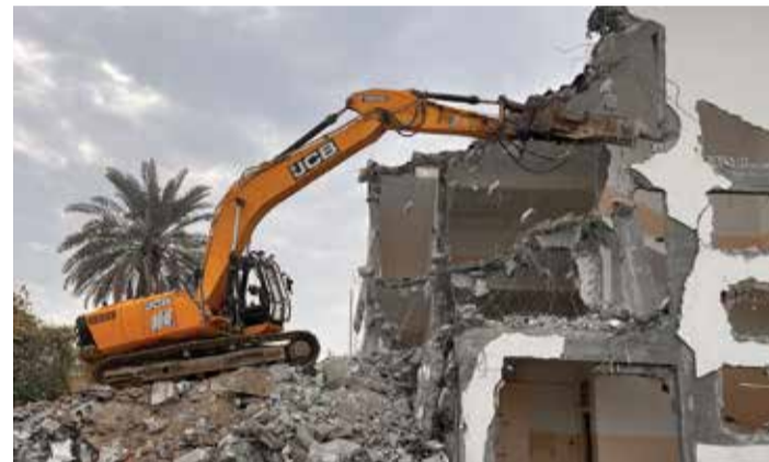
A building being bulldozed
