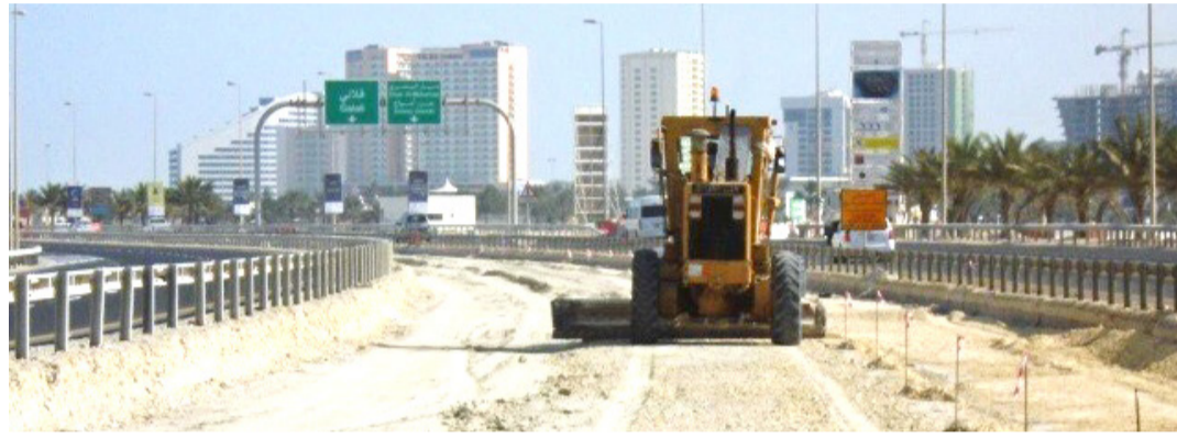
Work on the ring road is in progress
