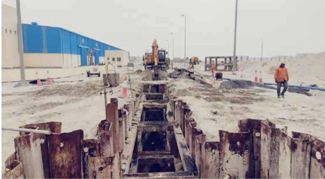
The main sewage water carrier construction work in progress
