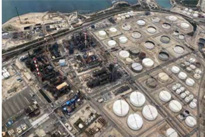
Storage tanks are seen at the Petroineos Ineos petrol refinery in Lavera, France, March
