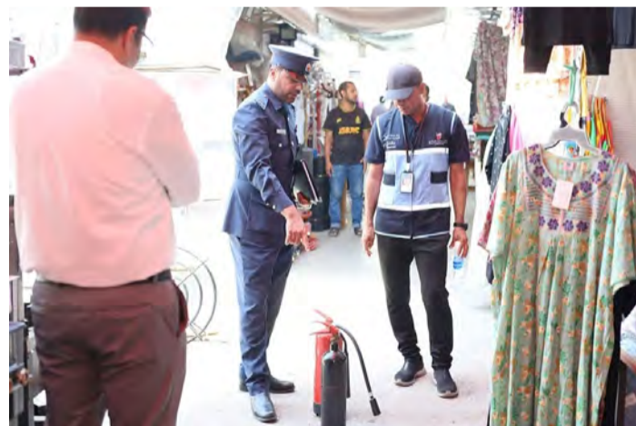
Fire extinguishers are checked for safety and effectiveness
