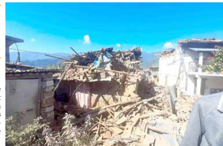
Damaged houses lie in ruins, in the aftermath of an earthquake at Pipaldanda village of Jajarkot district
