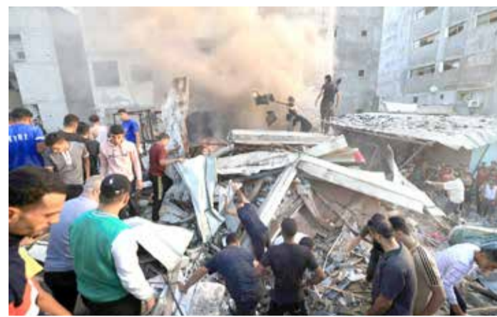
Palestinian search through the rubble of a collapsed building looking for victims and survivors following a strike by the Israeli military on Khan Yunis
