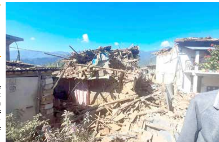
Damaged houses lie in ruins, in the aftermath of an earthquake at Pipaldanda village of Jajarkot district
