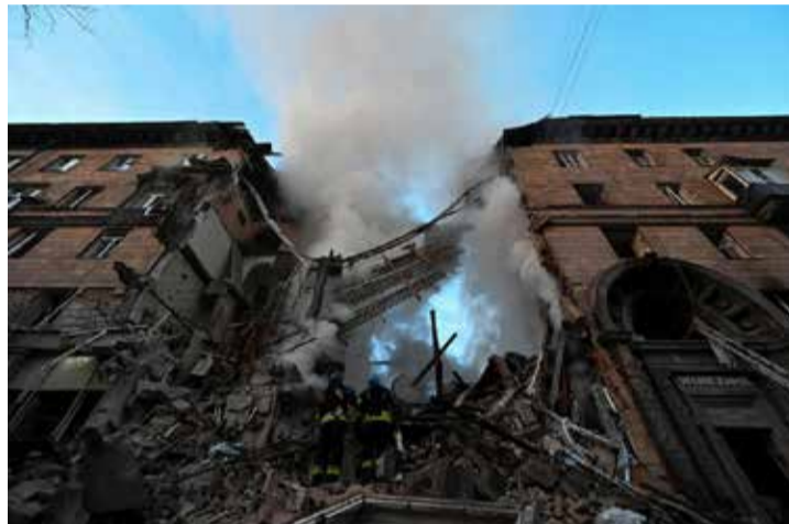
Rescuers work at a residential building which was heavily damaged by a Russian missile strike, amid Russia's attack on Ukraine, in Zaporizhzhia
