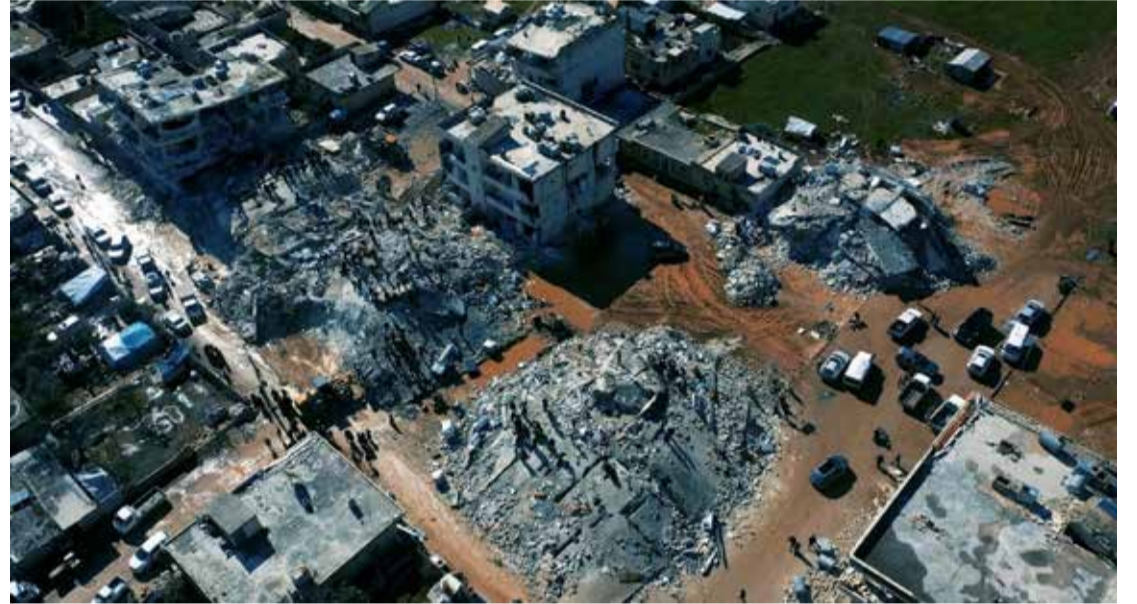
Damaged buildings and rescue operations are seen in the aftermath of the earthquake, in Aleppo, Syria February 7, 2023, in this screen grab taken from a social media video
