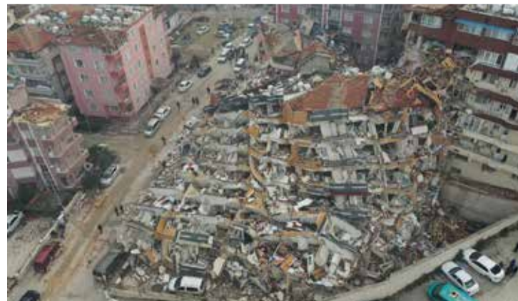
An aerial view shows damaged and collapsed buildings following an earthquake, in Hatay, Turkey
