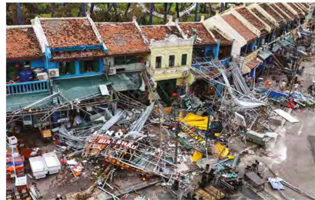
Damaged buildings and debris on a street after Super Typhoon Yagi hit Ha Long, in Quang Ninh province
