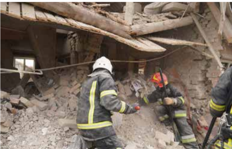
Emergency service workers search through the rubble for injured civilians in Ukraine's western Lviv Oblast
