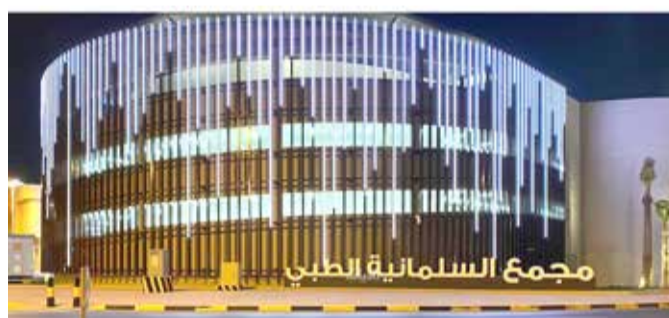
Some government buildings have already initiated steps to address the problems about security and safety
