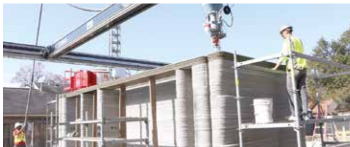
A 12-ton industrial 3-D printer is used to print concrete two-story home
