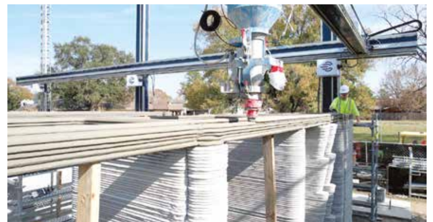
A construction worker watches as a 3-D printer lays concrete
