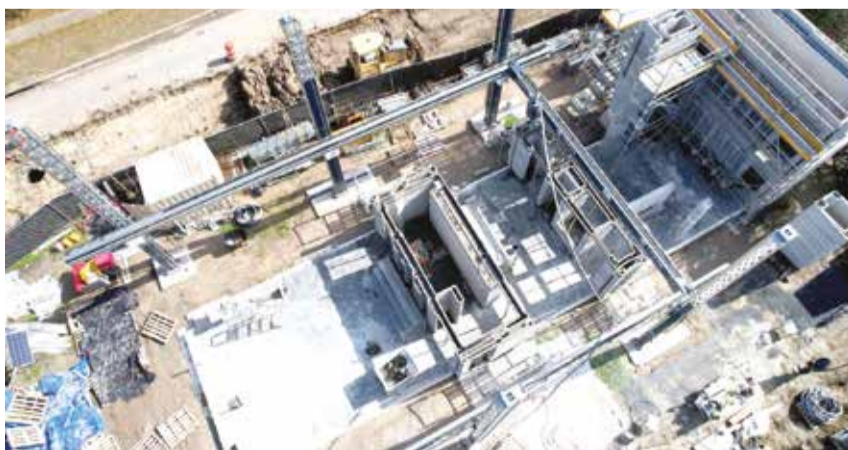
A 12-ton industrial 3-D printer is used to print concrete for the first 3-D-printed, two-story home under construction in Houston, Texas
