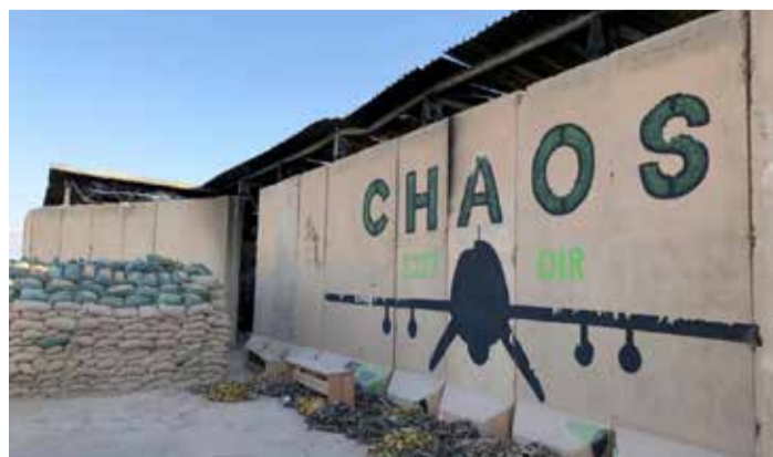
Blast walls of a sleeping quarters for US soldiers are seen at Ain al-Asad air base in Anbar province, Iraq
