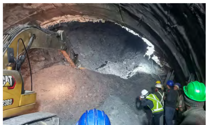
Rescue workers gather at the site after a tunnel collapsed in the Uttarakhand district of India's Uttarakhand state
