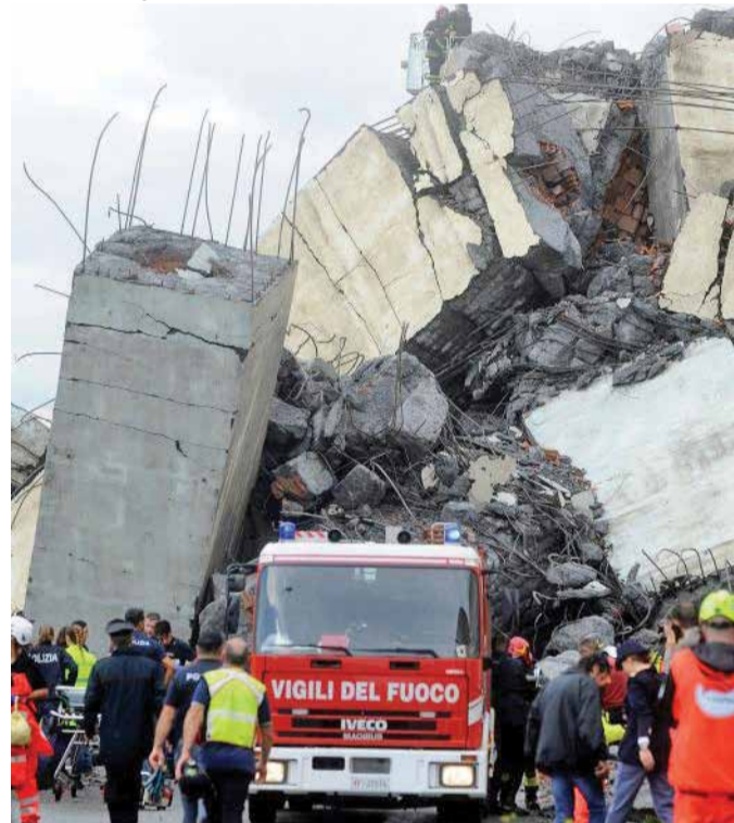
At least 35 people were killed yesterday when a giant motorway bridge collapsed in the Italian city of Genoa, with more feared dead in what one official described as an "immense tragedy". The collapse, which saw a vast stretch of the A10 freeway tumble on to railway lines in the northern port city, came as the bridge was undergoing maintenance work, and the country's deputy transport minister warned the death toll could climb further. See Page 13
