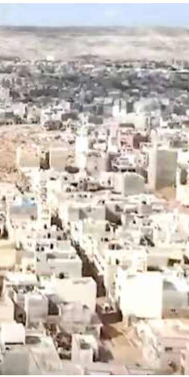
al view of a extensive damage in the wake
