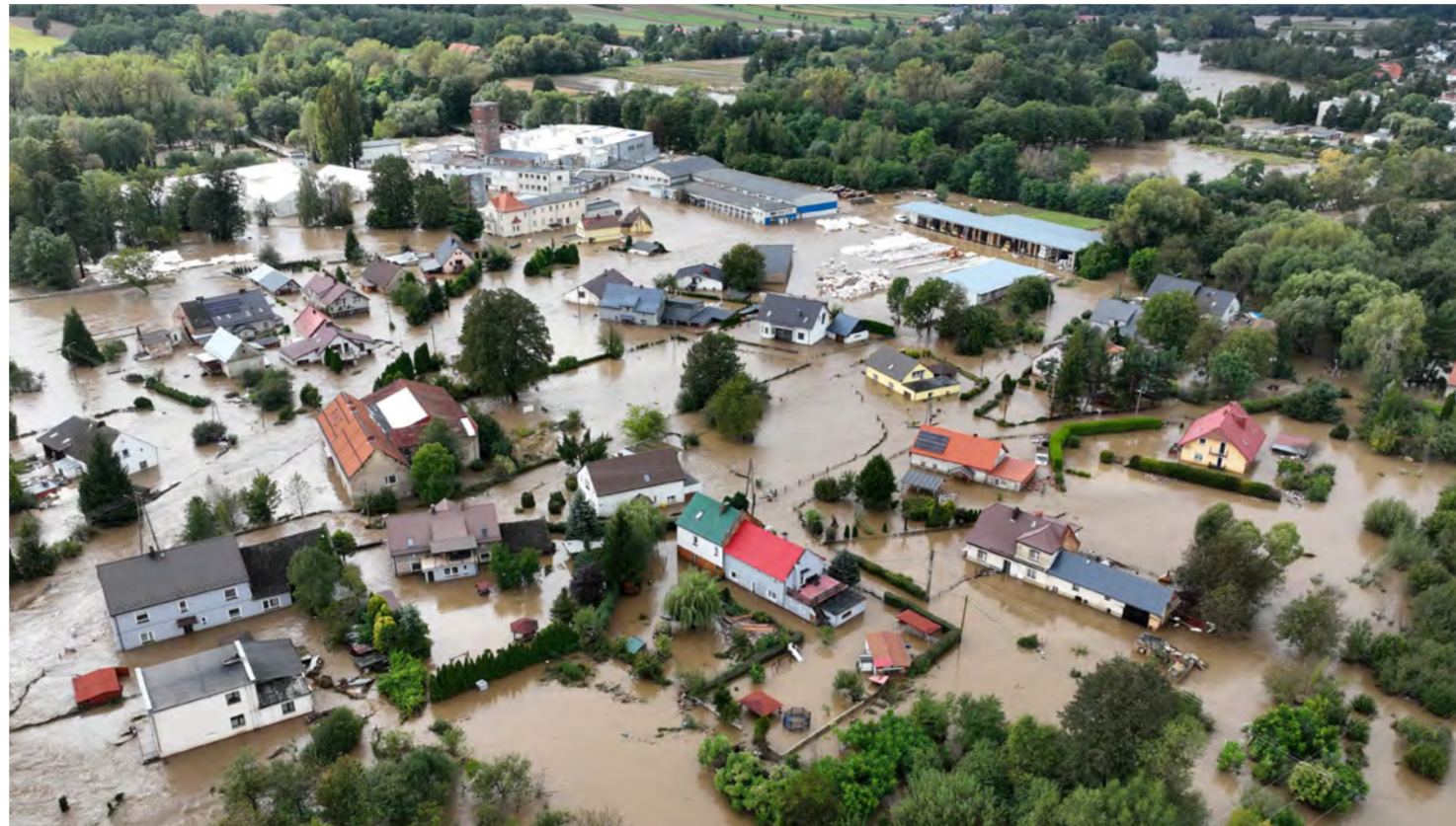
the flooded village of Rudawa, southern Poland
