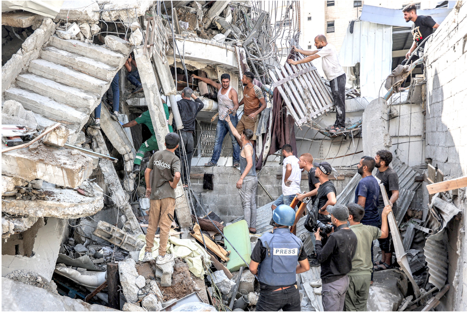
People gather outside a collapsed building as they attempt to extricate a man from underneath the rubble following Israeli bombardment in the Saffawi district in Jabalia in the northern Gaza Strip
