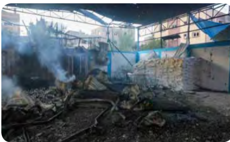
A damaged UNRWA food aid warehouse and distribution center due to Israeli strikes in Tall al-Hawa neighbourhood in southern Gaza City
