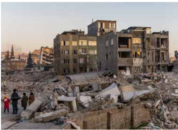
People look at damaged buildings and piles of rubble in the aftermath of a deadly earthquake in Kahramanmaraş
