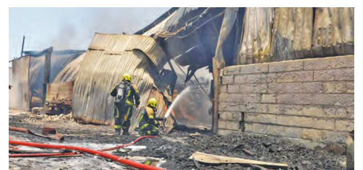
Firefighters battle flames to safeguard lives and property
