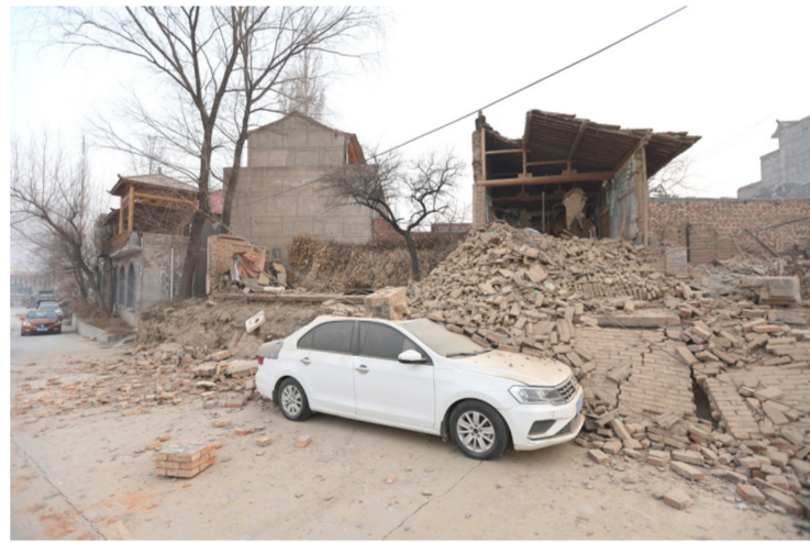
Collapsed buildings are seen after an earthquake in Dahejia, Jishishan County, in northwest China's Gansu province
