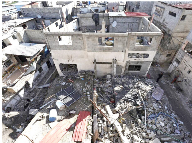
The rubble of a demolished house in the refugee camp in Tulkarm
