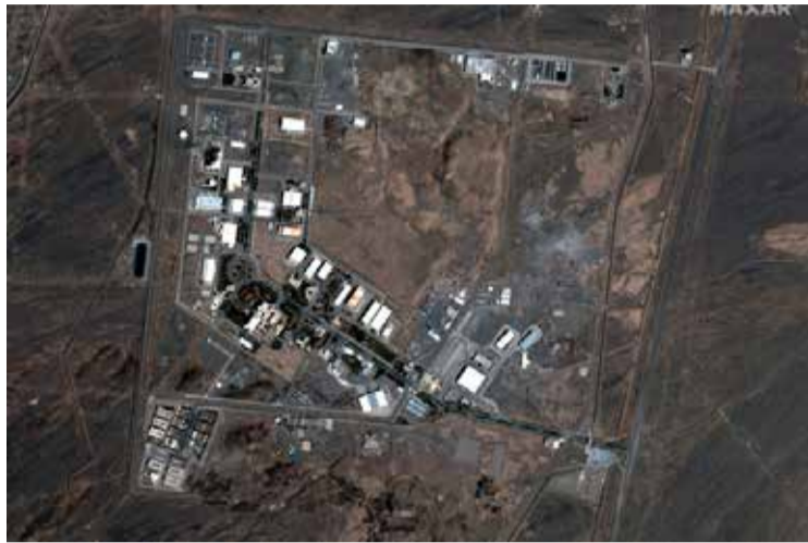
A handout satellite image shows a general view of the Natanz nuclear facility after a fire, in Natanz, Iran July. (file)
