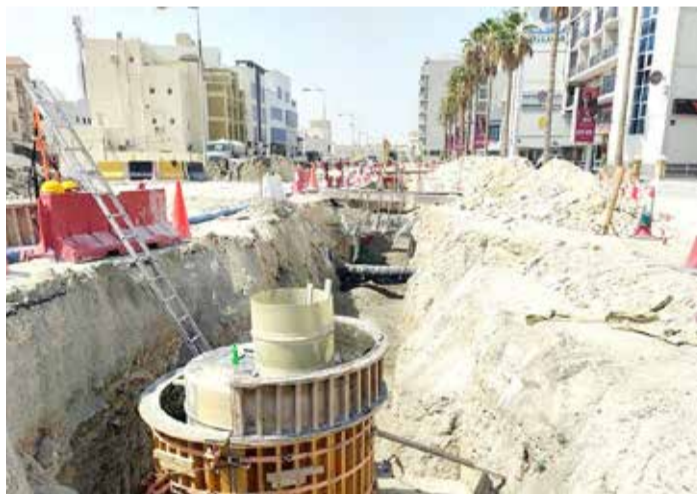
Work in progress on a new rainwater drainage network
