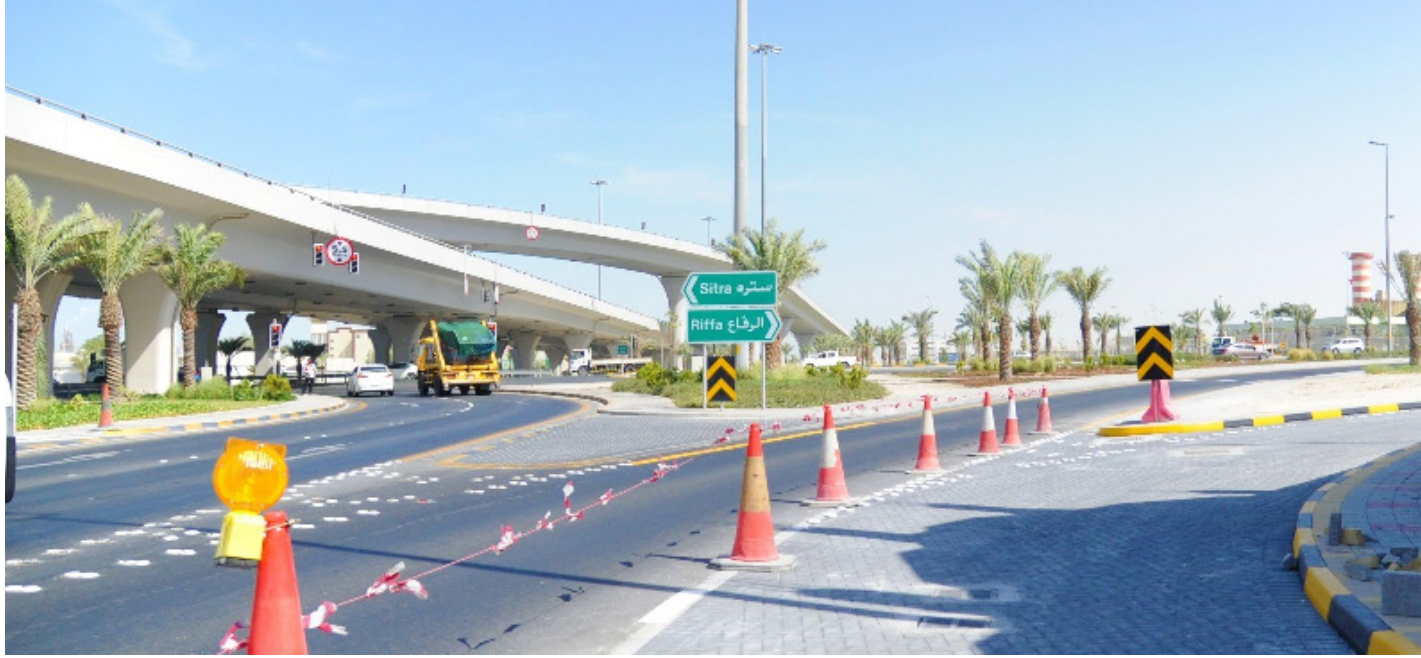
The projects offer solutions to traffic issues
