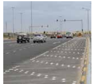
The road connecting Hunainyah Avenue to Al Muaskar Highway
