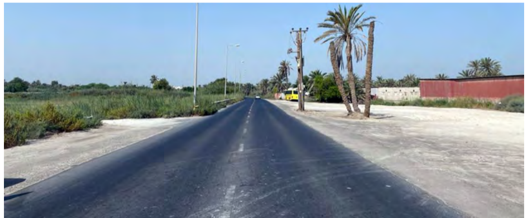
The Sar Avenue now provides safer and smoother flow of traffic
