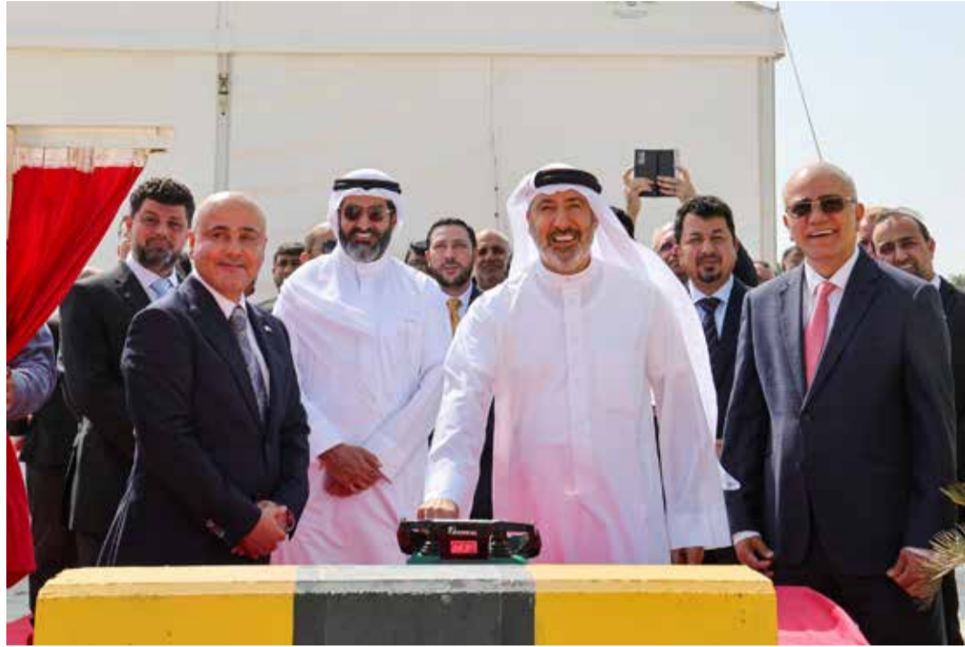
Shaikh Daij performs the First Concrete Pour for the foundation of Power Station 5 (PS5) Block 4 Project
