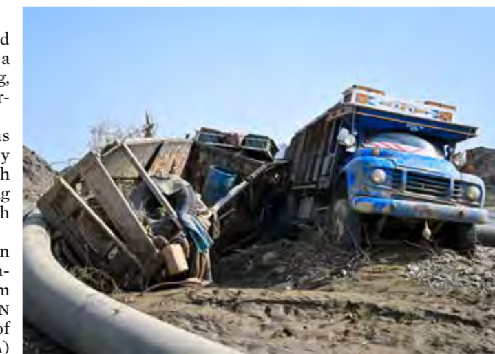
Damaged trucks buried in the mud after the collapse of the Arbaat Dam, 40km north of Port Sudan following heavy rains and torrential floods
