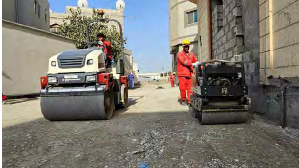
Resurfacing with new asphalt
