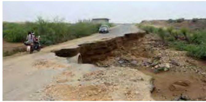
A motorcycle and a car drive through a road destroyed by flash floods in Yemen's northwestern Abs region in the Hajjah governorate
