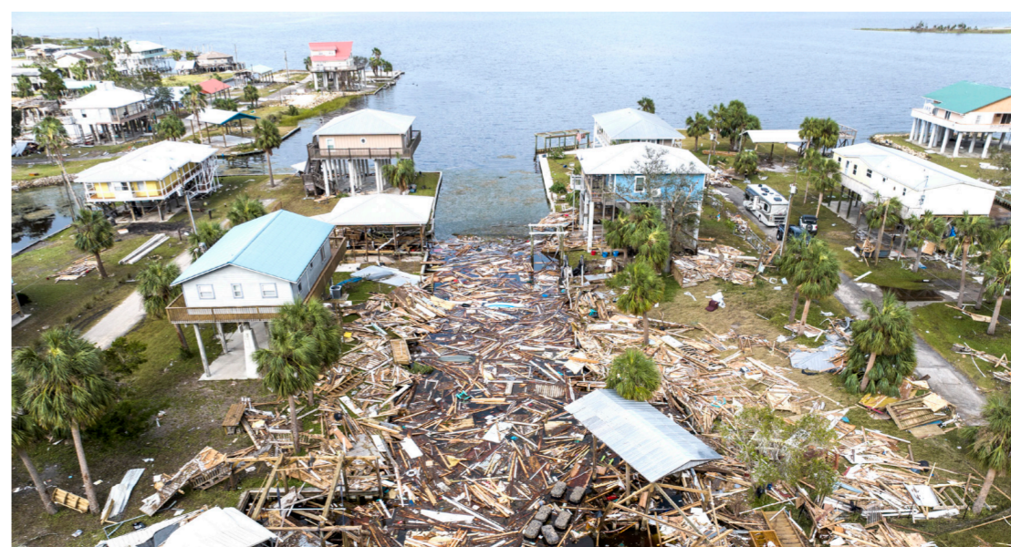
An aerial view of damaged houses are seen after Hurricane Helene made landfall in Horseshoe Beach, Florida
