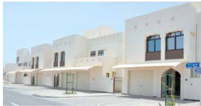
Rising concrete and material prices impact the construction industry
