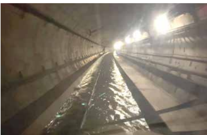
flooded water in a tunnel used by Eurostar trains, near Ebbsfleet International station in Kent, southern England
